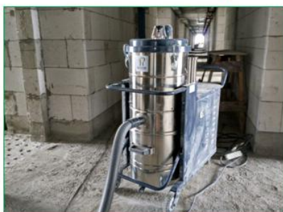
Construction job site
